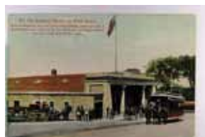
1371. Depot, Pearl Street, Tinted Printed Photo DB VF .. $15.00
