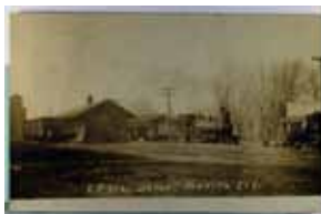
1356. Train Depot, Manito, Illinois, Real Photo, Used 1910 m cof Near VF .. $90.00
