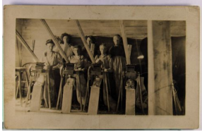
236. Women Working at Machinery, Real Photo w/ AZO P. C. back edge cr & m wear Near F-VF .. $25.00
