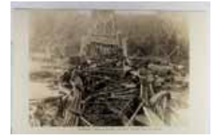
1595. Canada, Quebec, Disaster Scene, "Quebec Bridge After Collapse", Real Photo w/ AZO P.C. back m cor cr VF .. $15.00
