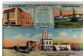
1328. Adv. King Tower Gas Station, Etc., Sioux City, Iowa, Curt Teich Pub. L VF .. $10.00
