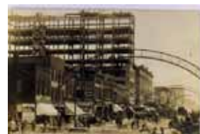
1530. Michigan, Flint, Real Photo, Used 1911 Near VF .. $15.00
