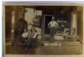
1573. Pennsylvania, Boynton?, Real Photo, Plumbing & Heating Co. Exterior m crs & album paper on back Near F-VF .. $75.00
