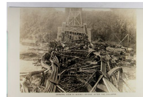
1595. Canada, Quebec, Disaster Scene, "Quebec Bridge After Collapse", Real Photo w/ AZO P.C. back m cor cr VF .. $15.00
