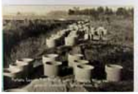
1516. Ohio, Bellefontaine, Real Photo, "Concrete Plant" VF .. $25.00
