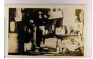
1525. South Dakota, Used Wolsey, "Clam Shack Interior", Real Photo m cor crs & wear F-VF .. $40.00
