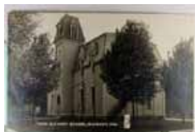
1478. Indiana, Elkhart, Real Photo w/AZO P.C. back, "East Elkhart School" VF .. $20.00
