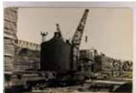
1468. California, Westwood, Real Photo w/ AZO P.C. back, "Red River Lumber Co." VF .. $40.00
