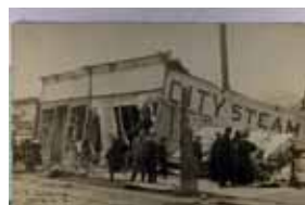
1505. Michigan, Cyclone Damage, Real Photo w/ AZO P.C. back m cor wear Near VF .. $25.00
