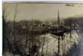
1554. Vermont, Wallingford, Real Photo, Used Same 1908 m wof F-VF .. $20.00
