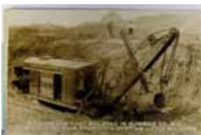
1533. North Dakota, McKenzie, Real Photo, "Building First Railroad", w/ Marion Steam Shovel, Used 1915 m cor wear F-VF .. $20.00
