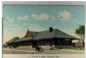
1351. Depot, Ashtabula, Ohio, Tinted Printed Photo DB m st & m cor wear Near VF .. $15.00
