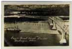
1476. Iowa, Dubuque, Real Photo w/Kruxo P.C. back, "Eagle Point High Bridge" VF .. $15.00
