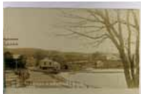
1491. Massachusetts, South Westport, "Hix Bridge", Real Photo w/AZO P.C. Back VF .. $20.00
