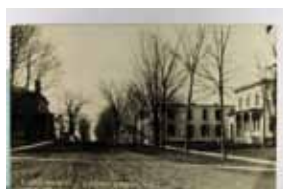
1519. New York, Central Square, Real Photo w/AZO P.C. back m cor wear VF .. $35.00
