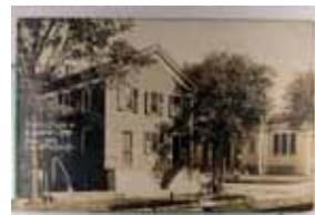
1439. Indiana, Elkhart, Real Photo m cor wear F-VF .. $15.00
