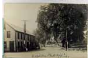
1448. Massachusetts, Dighton, Real Photo, Post Office Incl. in Street Scene m wof Near VF .. $20.00
