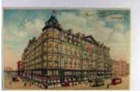
811. Hold to the Light, Die Cut, J. Koehler Pub. #2409, "Palmer House, Chicago, Illinois", Used 1915 DB VF .. $30.00
