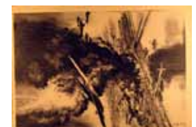
1293. W.W. II German pub., Fabrikund Hafenanlagen, CTO 1943 m cor wear F .. $50.00
