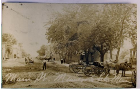
1457. Minnesota, Used Wells, Real Photo w/ AZO P.C. back, "Main St." cof & m cor cr Near F-VF .. $15.00
