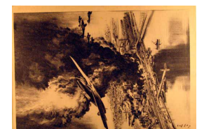
1293. W.W. II German pub., Fabrikund Hafenanlagen, CTO 1943 m cor wear F .. $50.00
