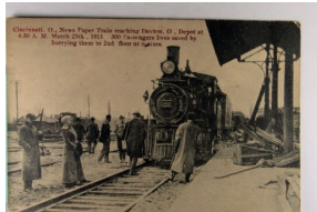
1382. Train Wreck into Depot, Dayton, Ohio, Photogravure, Dated March 25th, 1913 DB m cor wear Near VF .. $25.00
